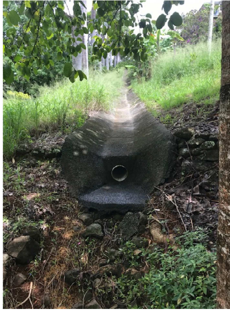
Figure 1: Photo of existing stormwater pipe & concrete drain
