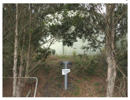
Figure 12: Fire Fighting Outlet at SWERF & Water Storage Tank.
