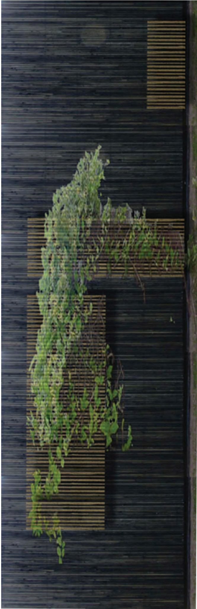
BLOCK 3A SOUTH WALL ELEVATION - TIMBER PANELS ATTACHED TO WALL. CREEPERS AT 3 LOCATIONS
