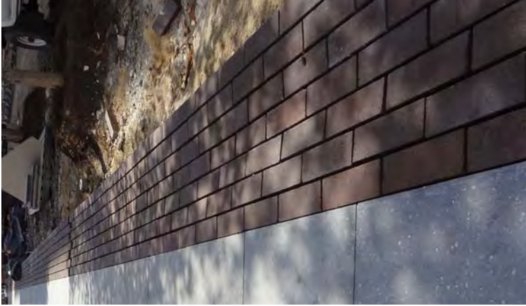
CHIPPENDALE GREEN BRICK DISH DRAIN
