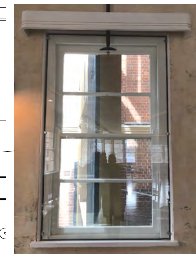
Acoustic and thermal internal glazing to all windows to existing heritage approved details.
