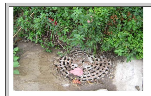
PHOTO P11 Grated Stormwater inlet pit.
