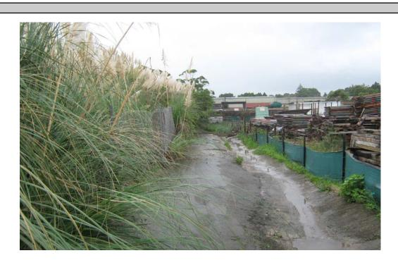
PHOTO P14 View north of concrete lined channel with silt fencing on right.
