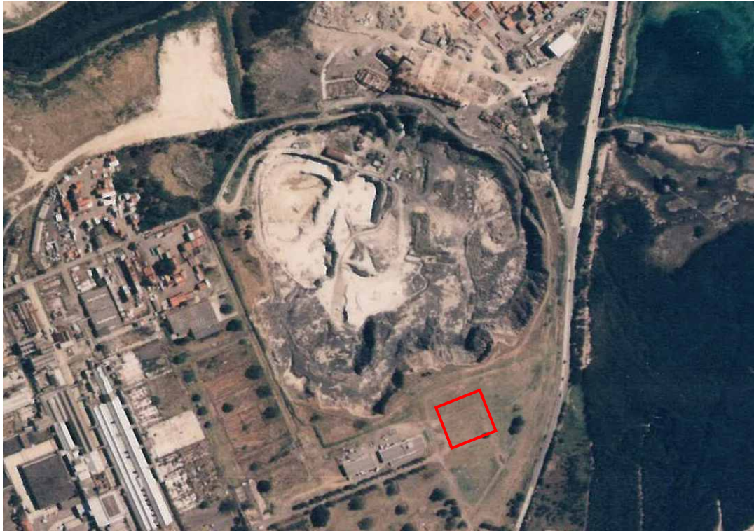
Photo 7: Aerial photo from 1991
