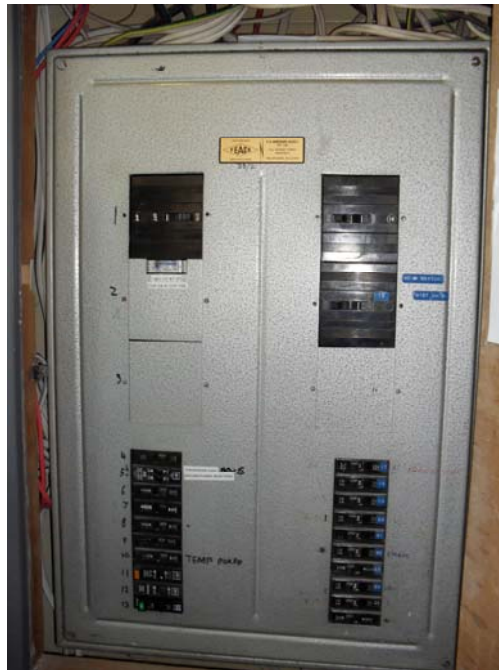
Existing non-compliant distribution board (to be replaced)
