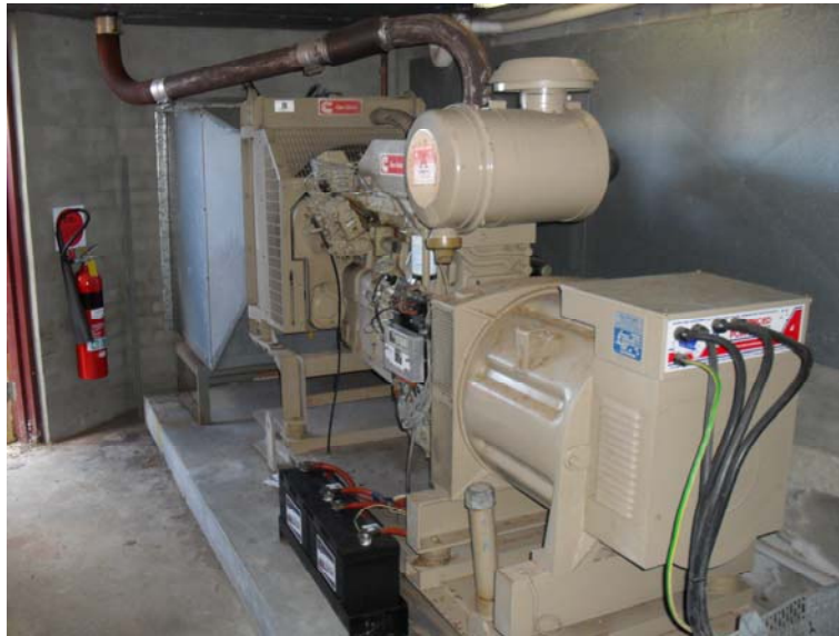
Existing 190kVA diesel generator
