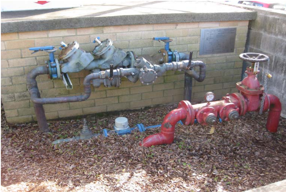
Incoming cold water supply and backflow prevention device
