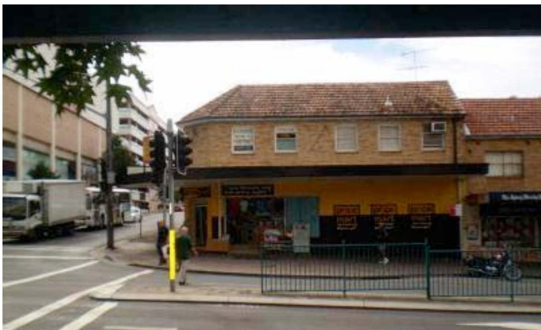
Figure 7. View of the Site fronting Kiora Road
