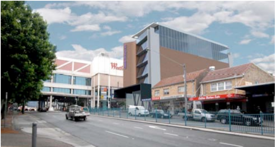
Figure 12. Visualisation of the Building Looking North along Kiora Road
