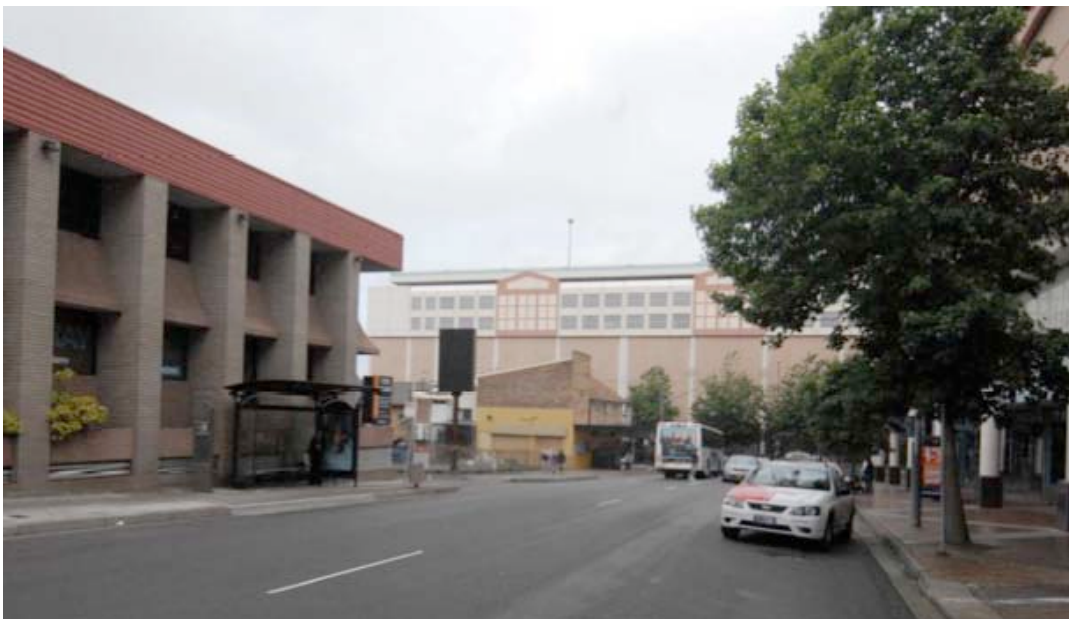
Figure 4. View of Urunga Parade Looking West
