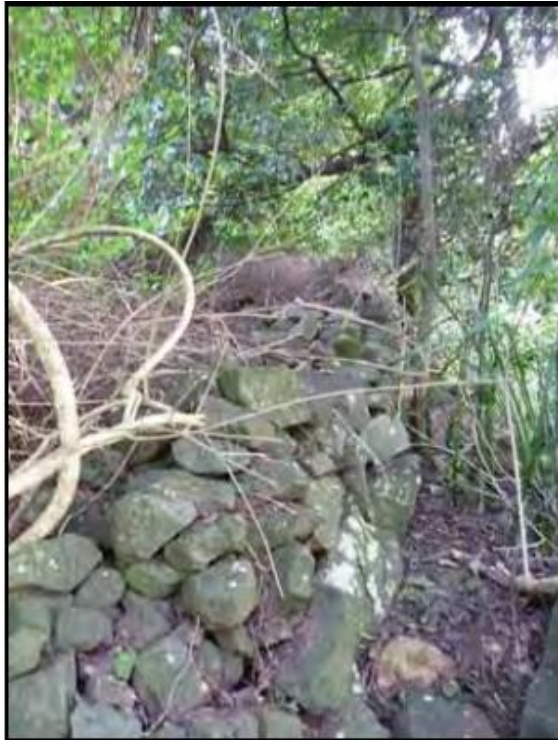
These show use of the A frame technique, but some loss of coping stones. It is reasonably intact
