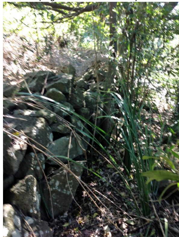
These basaltic rocks are harder to fit than weathered latite and have not been well graded; nor do they tilt inwards.
