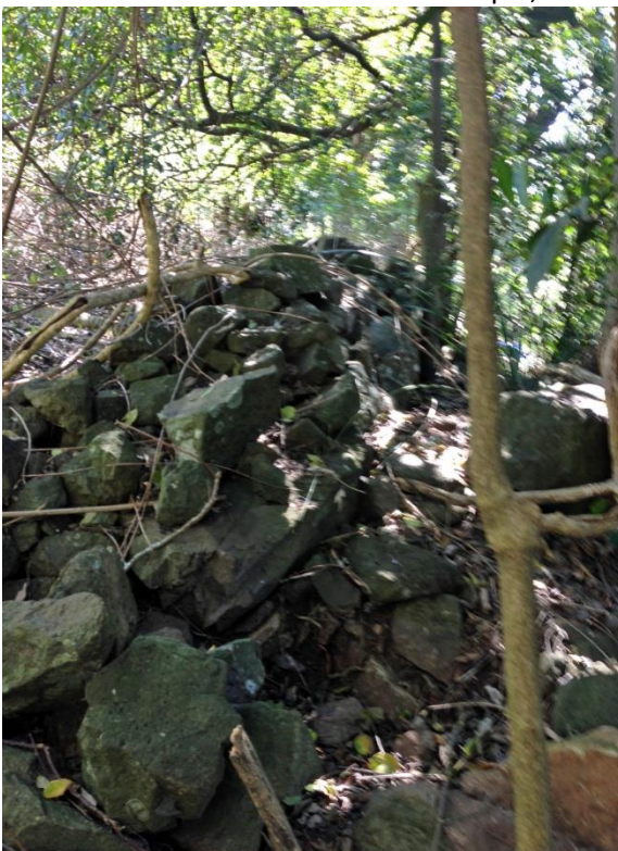
This shows poorly selected and fitted basaltic stones, resulting in some collapse, to which adjacent vegetation is contributing
