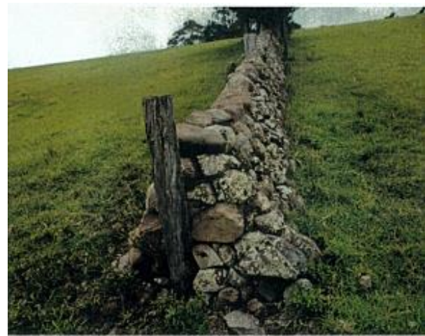
A well (re)constructed, A-Frame wall near Kiama
