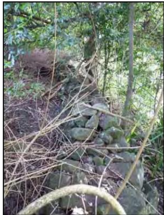
These show use of the A frame technique, but some loss of coping stones. It is reasonably intact
