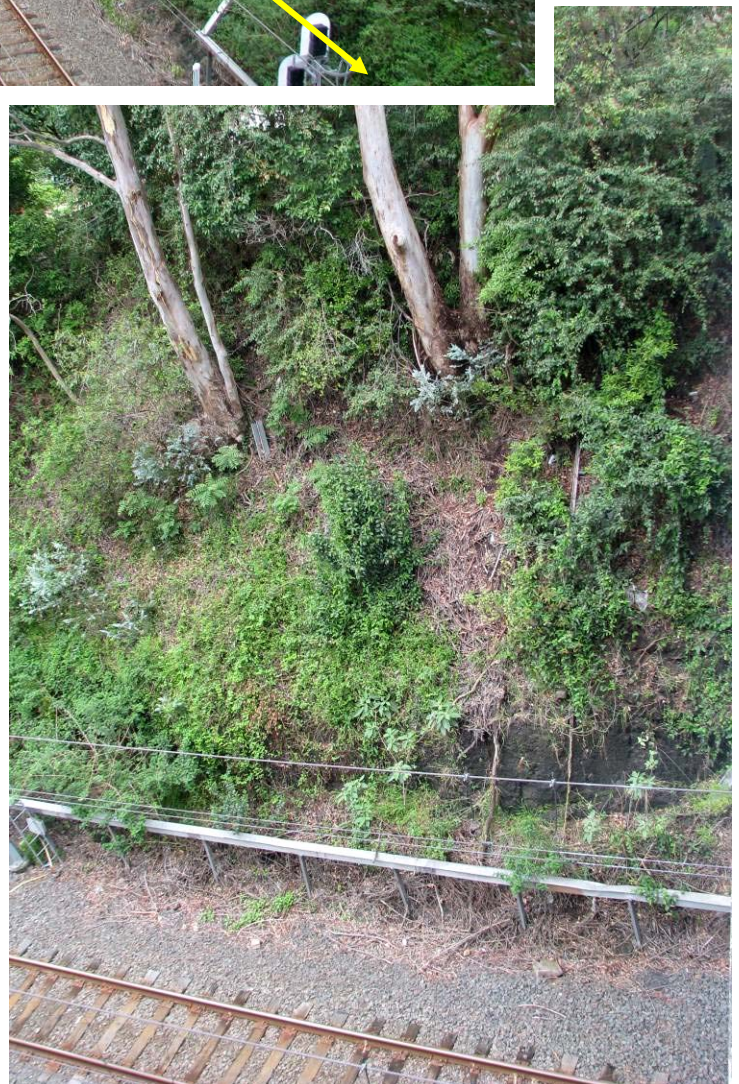
PHOTOGRAPH 2: View of cut batter on south-eastern side of Beechworth Road bridge, showing shale exposed at base of cutting.
