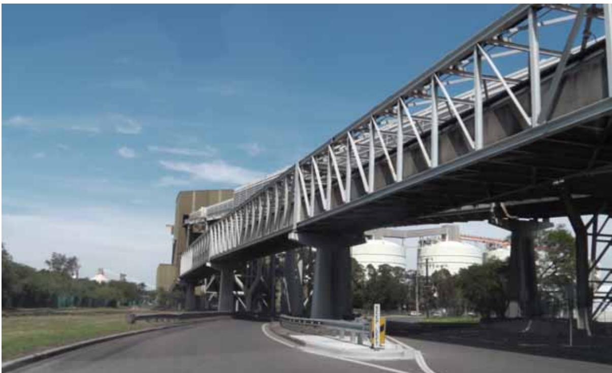
Photograph 2.6 KCT outbound conveyors built over the local road section of Cormorant Road
