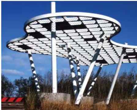
Pergola sructure to town square
