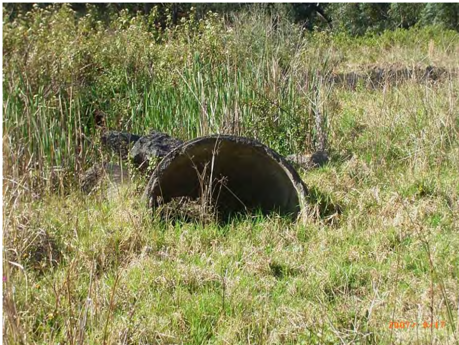
Partially exposed concrete pipe on edge of drainage swale in main benched area of former quarry/landfill.
