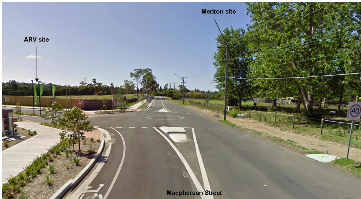
Figure 6: Roundabout at the intersection of Macpherson Street, the ARV site and the Stage 1 development (Source: Google Maps, 2012)
