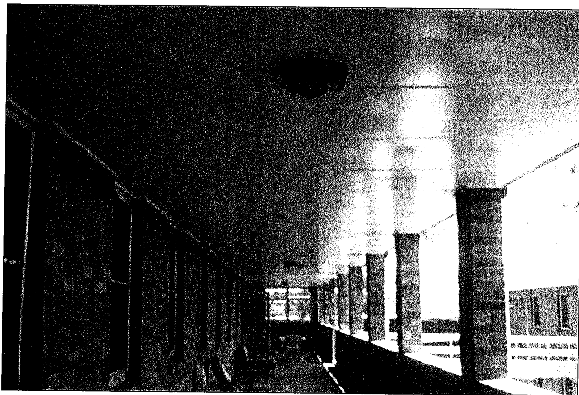
Photograph No. 93: Suspected Asbestos Cement Sheet to Verandah Ceiling Lining
