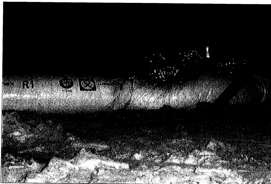
Photograph No. 14: SMF in Plastic Insulation to Flexible A/C Ducts
