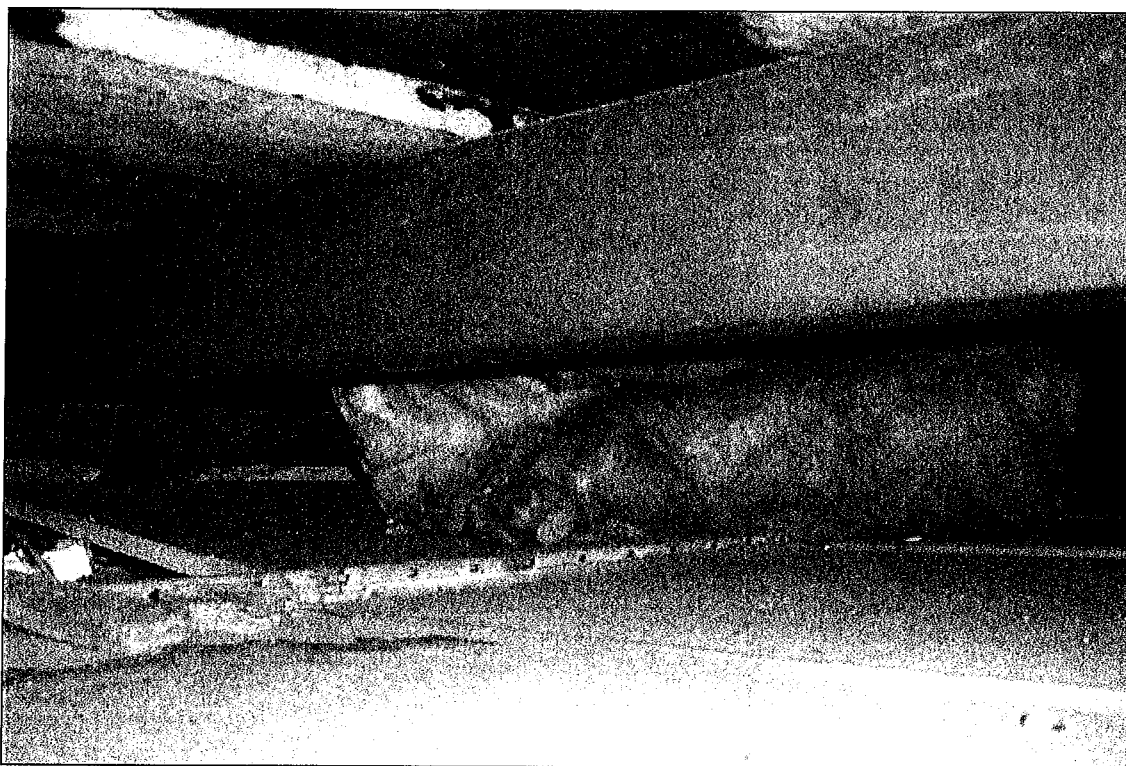
Photograph No. 123: SMF Batts in Ceiling Space
