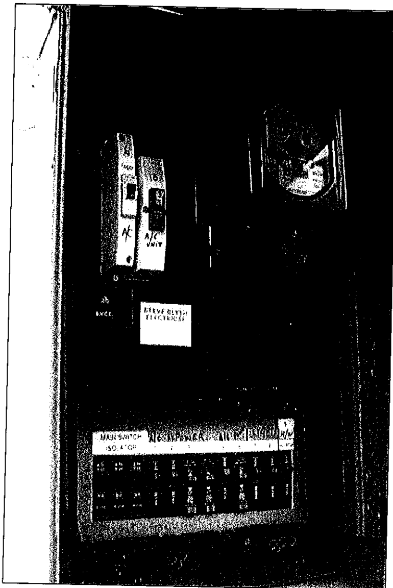
Photograph No. 172: Suspected Zelnite Backing Board to Electrical Switchboard
