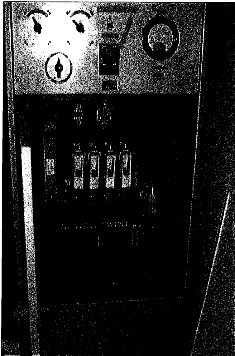
Photograph No. 83: Suspected Zelnite Board to Old Switchboard in Basement Below Children's Ward
