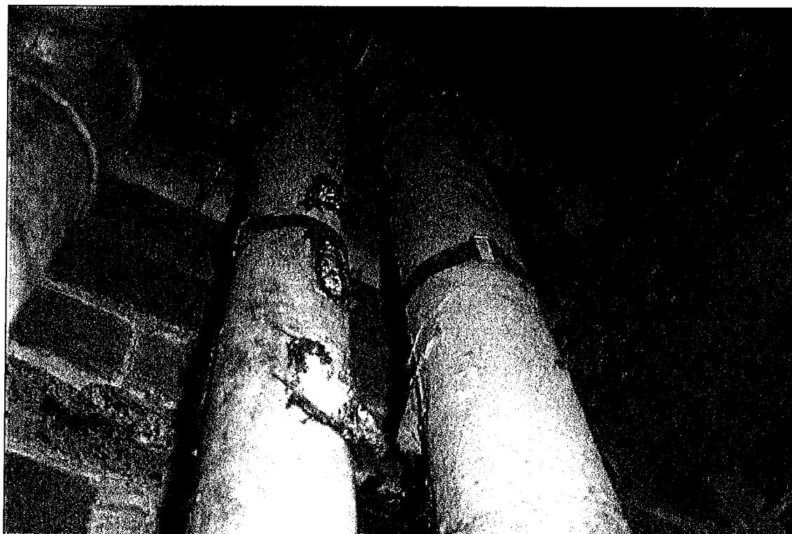
Photograph No. 97: Suspected Asbestos Insulated Pipes in Laundry Riser (Note Poor Condition)
