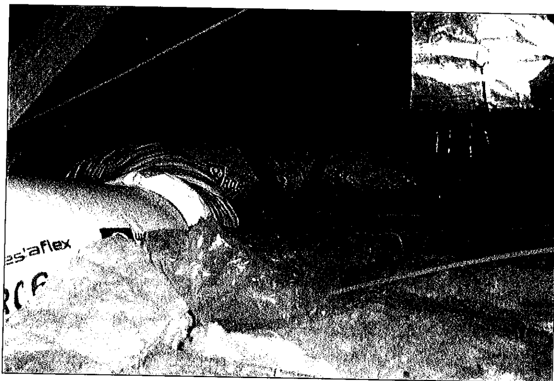
Photograph No. 157: Flexible A/C Ducts in Ceiling Insulated with SMF in Plastic
