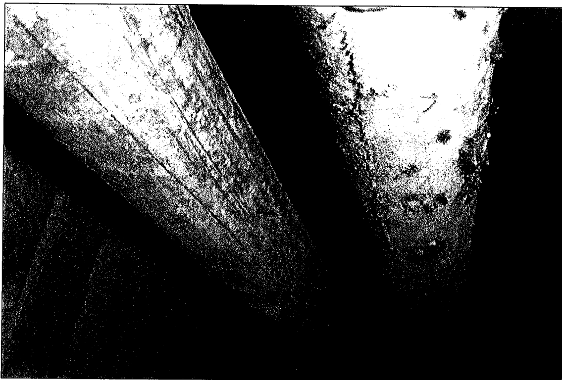
Photograph No. 95: Suspected Asbestos Insulated Pipe in Cleaners Room Looking Down Riser
