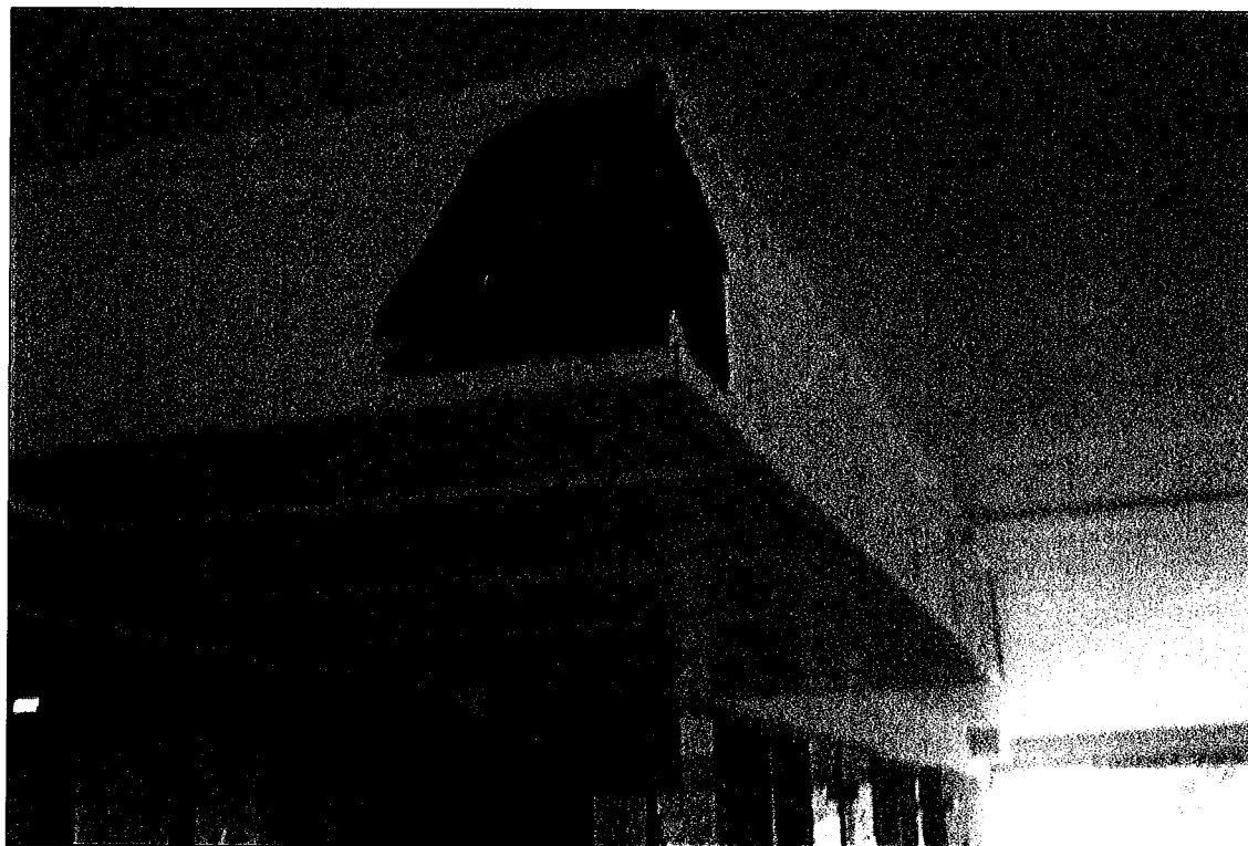
Photograph No. 117: Suspected Asbestos Cement Awning and Bulkhead at Entry (Note Damage)
