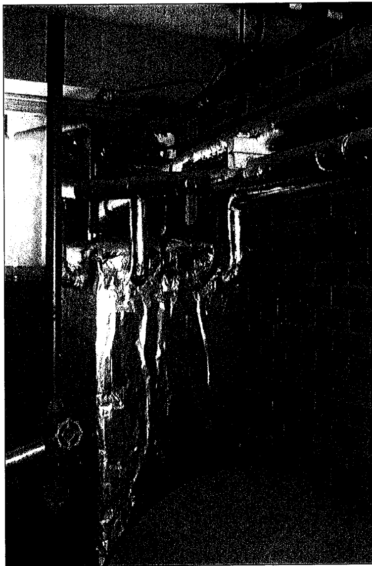
Photograph No. 81: SMF / Foil Insulation to Calorifier - Plant Room 7
