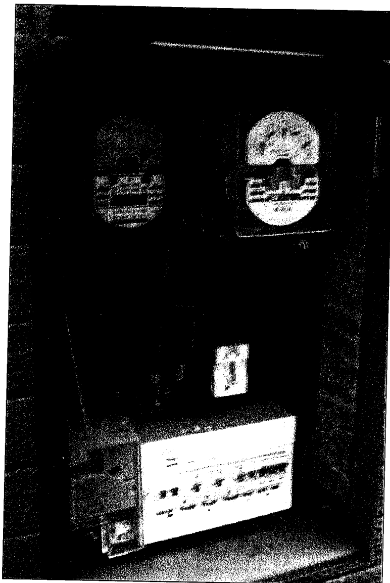
Photograph No. 3: Suspected Zelnite Backing Board in Electrical Switchboard
