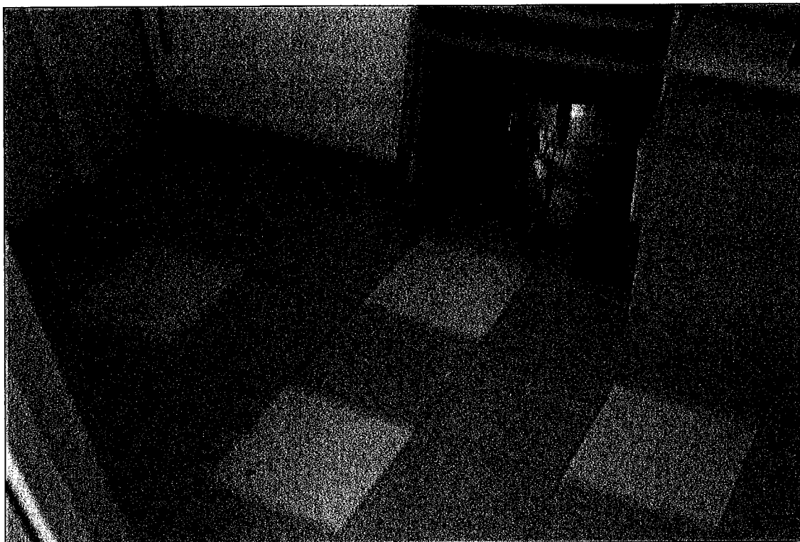
Photograph No. 7: Asbestos Vinyl Tiles to Laundry Floor
