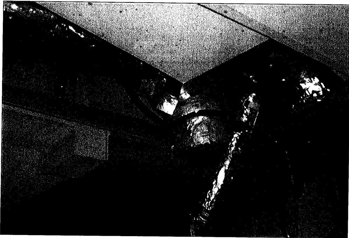
Photograph No. 52: Old Hot Water Steam Pipes in Tunnel Ceiling Space Insulated with SMF in Foil
