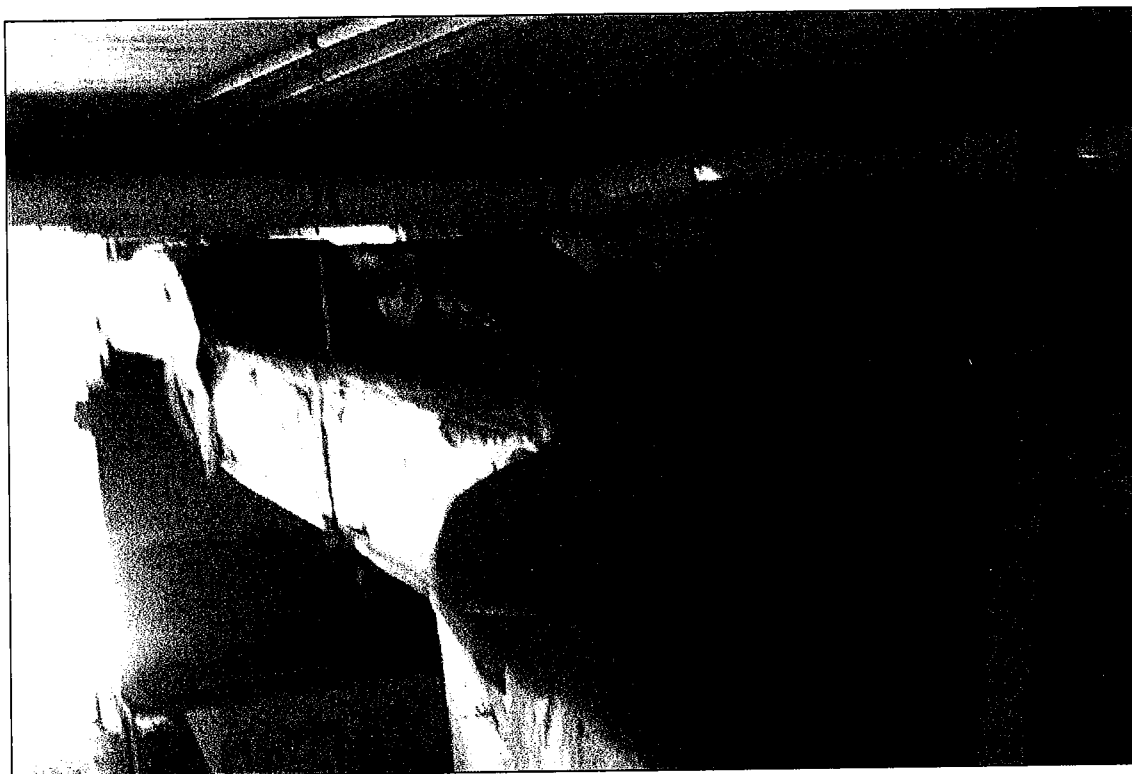
Photograph No. 104: SMF / Foil Insulation to A/C Ductwork in Plant Room
