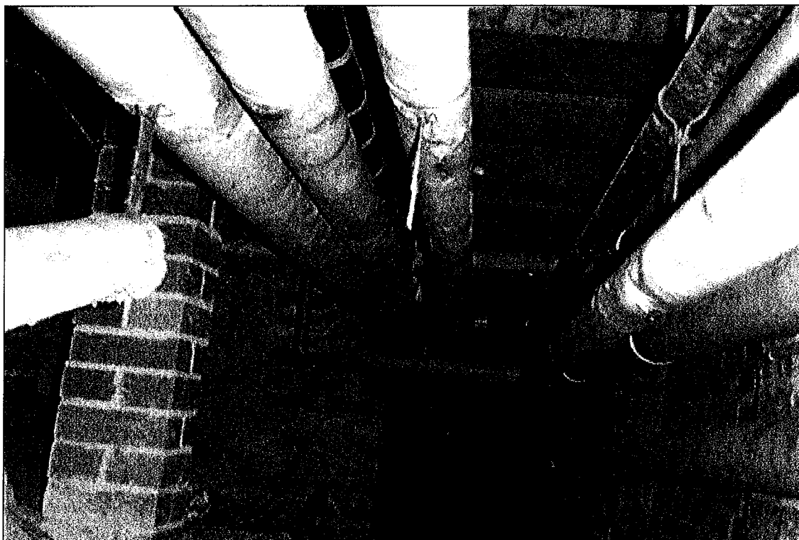
Photograph No. 113: SMF Insulated Pipes in Sub-Floor Area
