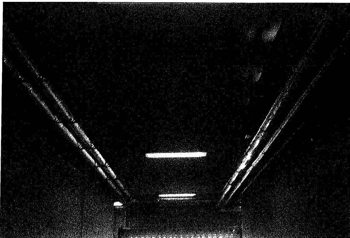
Photograph No. 56: Corridors - Hot Water Pipes Insulated with SMF in Foil
