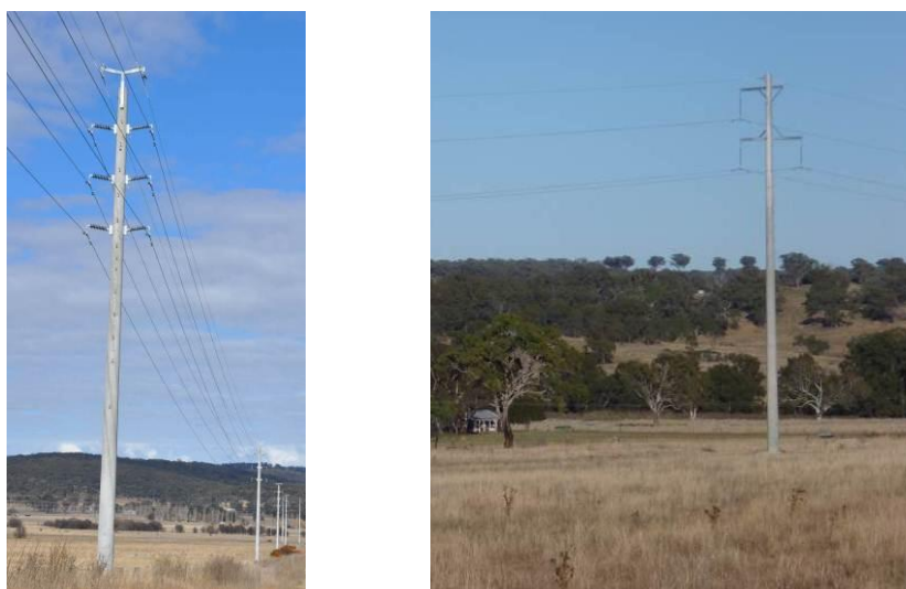
Figure 3-1 Existing double circuit & single circuit 132kV powerlines near the wind farm site
