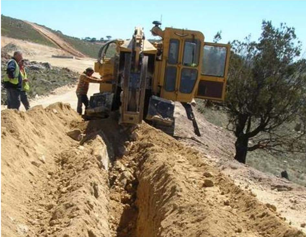
PLATE 3.5 – EXAMPLE OF UNDERGROUND CABLE TRENCH FOR 33KV BEING EXCAVATED
