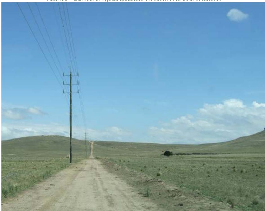
PLATE 3.2 – EXAMPLE DOUBLE CIRCUIT 33KV OVERHEAD TRANSMISSION LINE.
