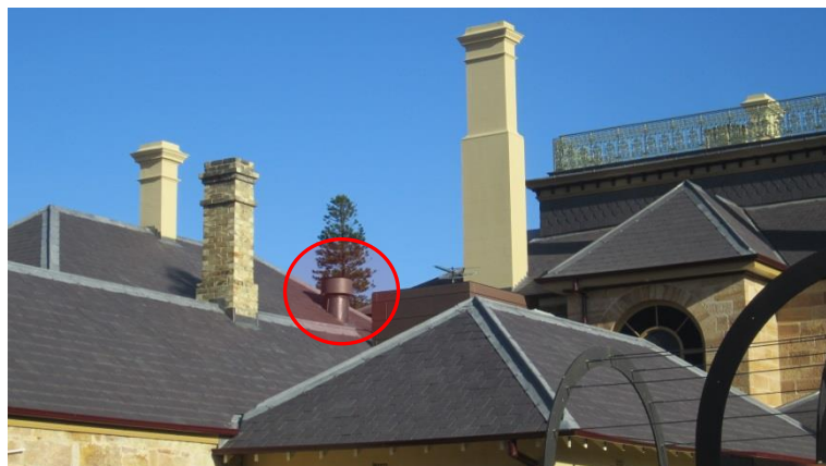
Figure 6: New kitchen exhaust fan within the red circle (Graythwaite building)
