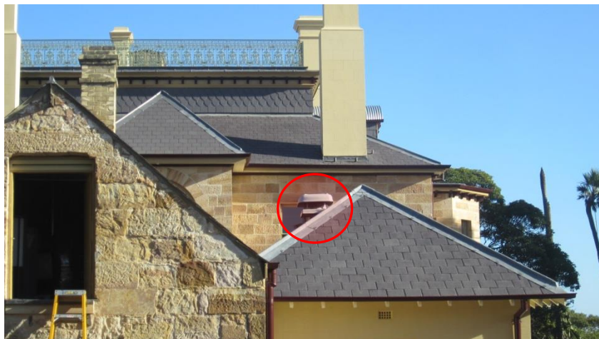
Figure 6: New kitchen exhaust fan within the red circle (Graythwaite building)
