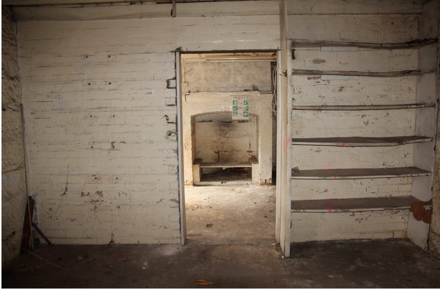
Figure 5 The existing opening between rooms G19a and G19b which is proposed to be widened. Source: TKD Architects, 2013.
