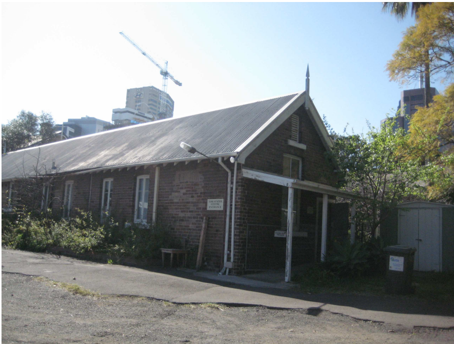
Figure 9 The c1950s or 60s skillion-roofed verandah and subsequent entry opening, proposed to be removed.
