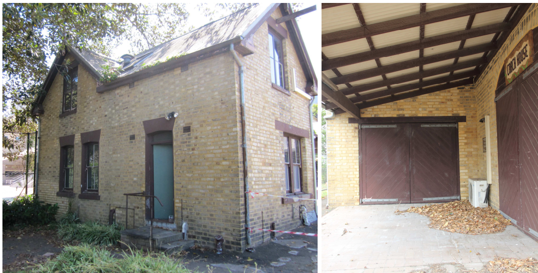
Figure 8 The Coach House's non-original steps and doorway on the western elevation of the building and the c1970s timber ledged and braced door in the verandah; both of which are proposed to be removed and replaced as part of the Stage 1 Works. Source: TKD Architects 2010 and 2013.
