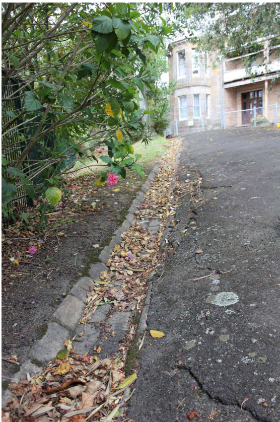
Figure 3 Remnant 1890s brick drain along the upper driveway. Source: Tanner Kibble Denton Architects, 2013.
