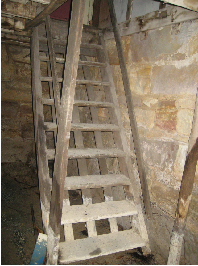
Figure 4 Non-original timber-framed basement stairs proposed to be replaced. Source: Tanner Architects, 2010.
