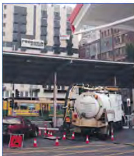
Cleaning of an RSF 4000 by eductor truck
