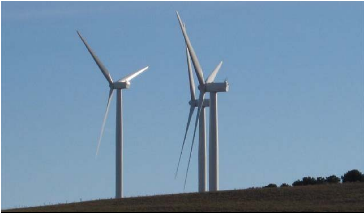
Figure 68: Blade glint is not significant on the blades of modern turbines due to the non-reflective paint that is used on the surface of the blades
