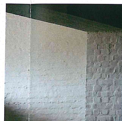
Example of type 4 finish - Bagging with integral colour in the render.
