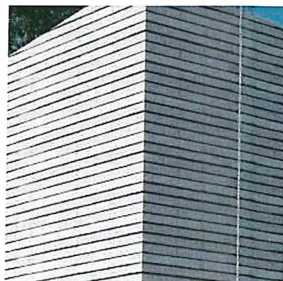
Example of type 2 bond - Raked horizontal joints with flush perpend
