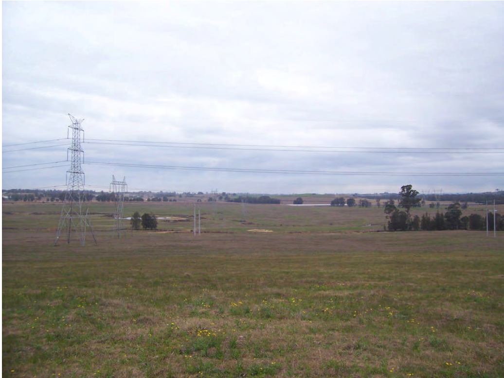
Photograph 03: Looking south from the northern portion of the site.
