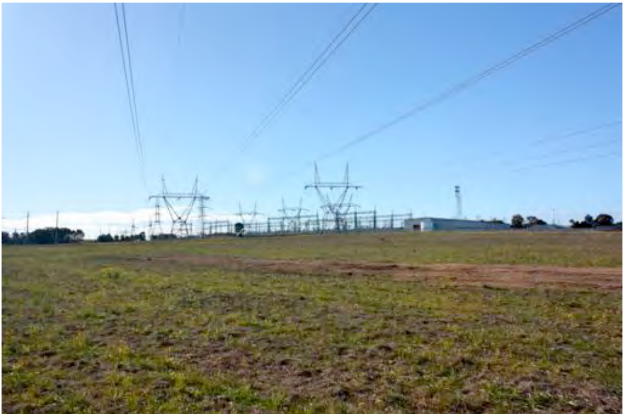
Photo 2 Looking east from Photo Point 1 towards the TransGrid substation. The southeastern part of the Stage 1 Project Application site is located in the right of the photo.
