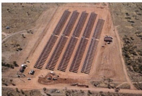
Figure 3. View of 1 MW Uterne Solar Farm, a tracking solar farm installed in Alice Springs
