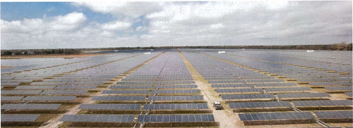
Figure 6 provides an example view of tracking array blocks in operation.
