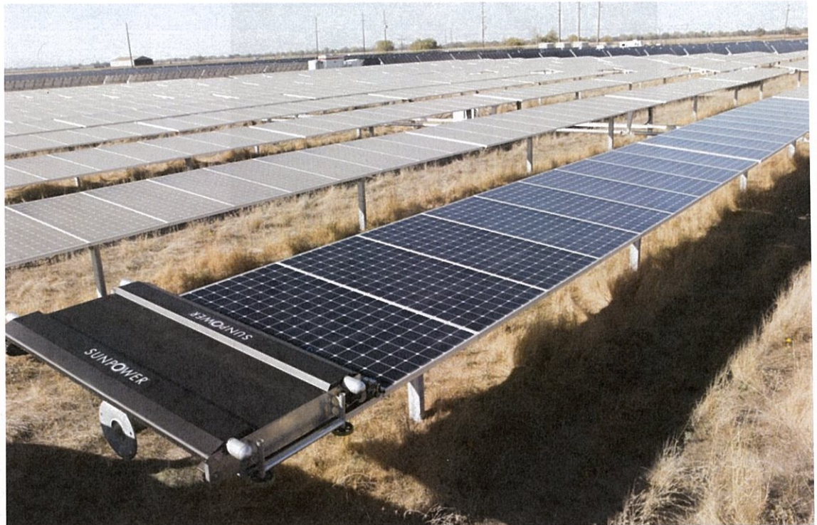
Figure 2. C1 Solar Tracking System – Position in Middle of Day (flat with respect to horizon)
