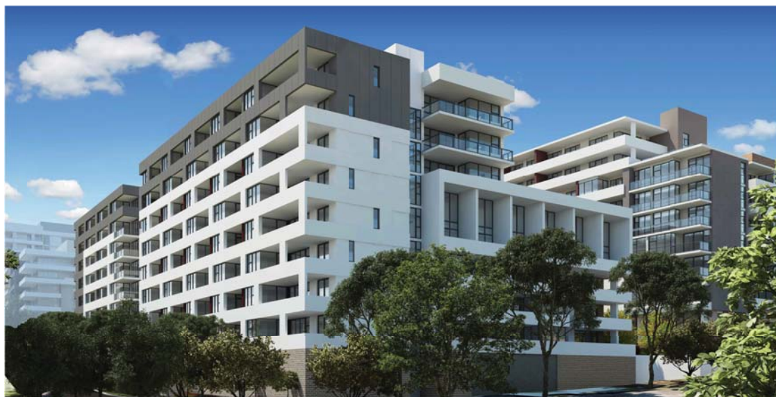
6 VIEW FROM NORTH-WEST CORNER NTS
