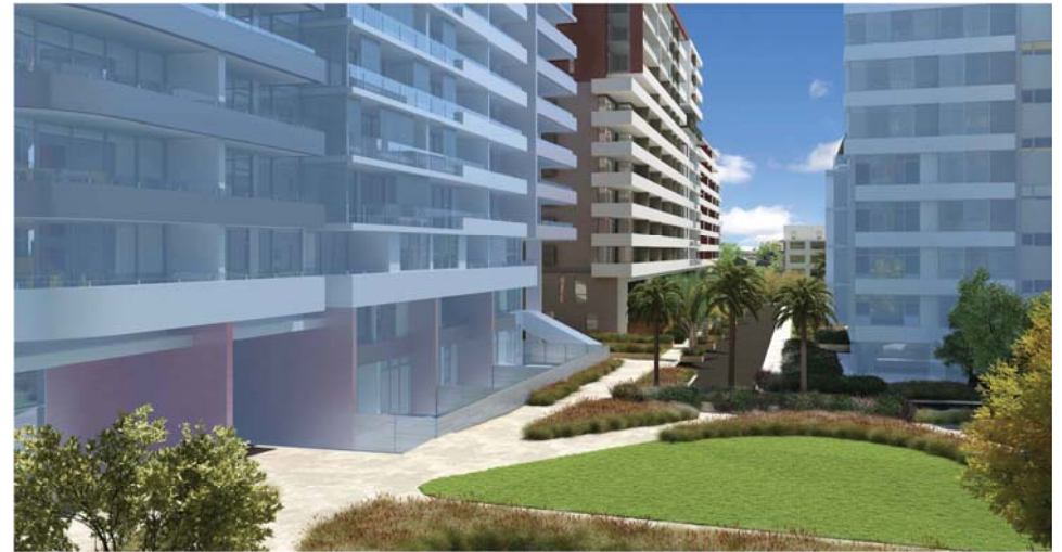
7 INTERNAL VIEW LOOKING WEST NTS
