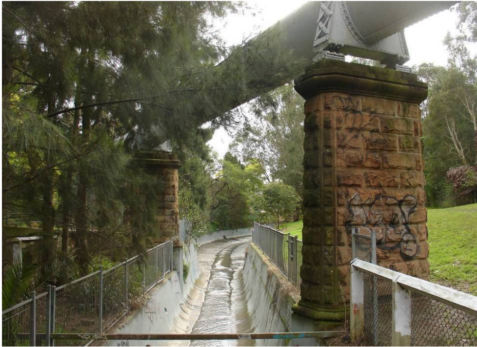
Figure 5.26 Lewisham Sewage Aqueduct, over the Hawthorne Canal, note relatively narrow interval between sandstone piers.
