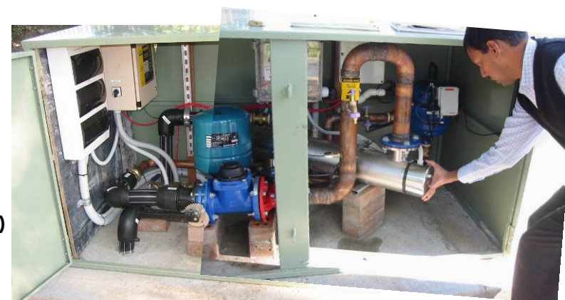
Example of a stormwater pump and treatment system for a harvesting scheme at Ryde Park
