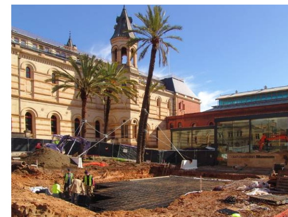
Modular plastic stormwater tank under construction at the South Australian Museum
