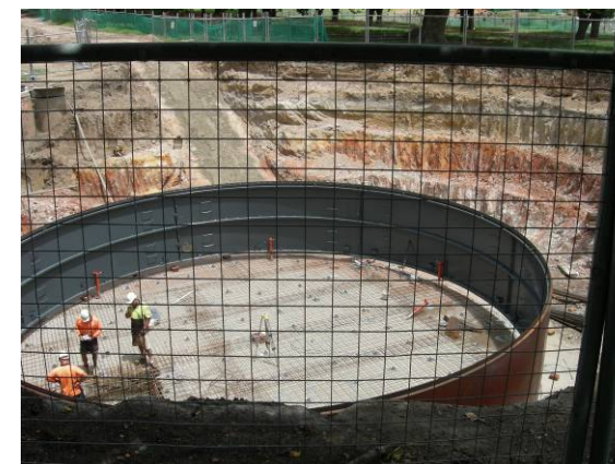
200 kL concrete stormwater tank under construction at Prince Alfred Park in Sydney
