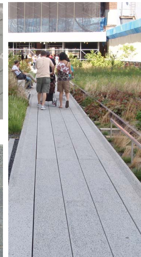
Type 4: Platform : example of Precast concrete units Highline project, New York
