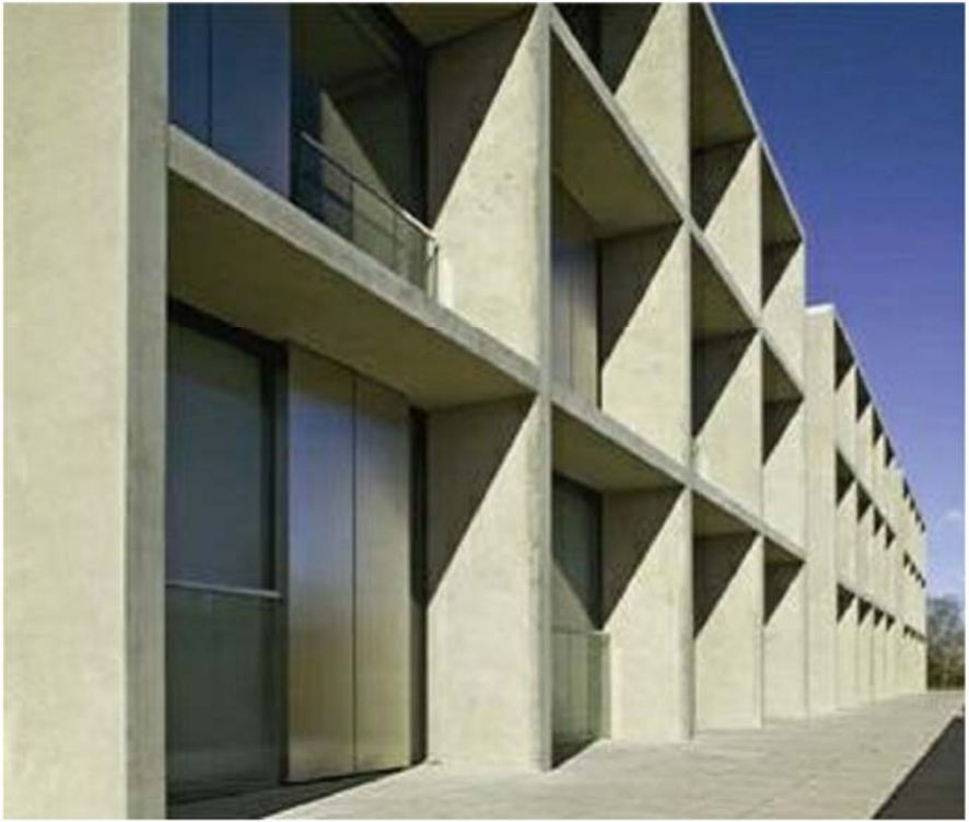
VERTICAL FINIS - PRECAST CONCRETE PANELS (VF)
