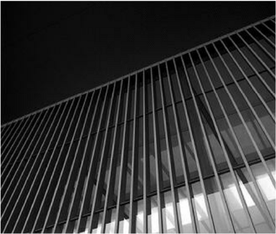
VERTICAL EXTERNAL SOLAR SHADING ELEMENTS, POWDERCOATED ALUMINIUM (DARK COLOUR)
