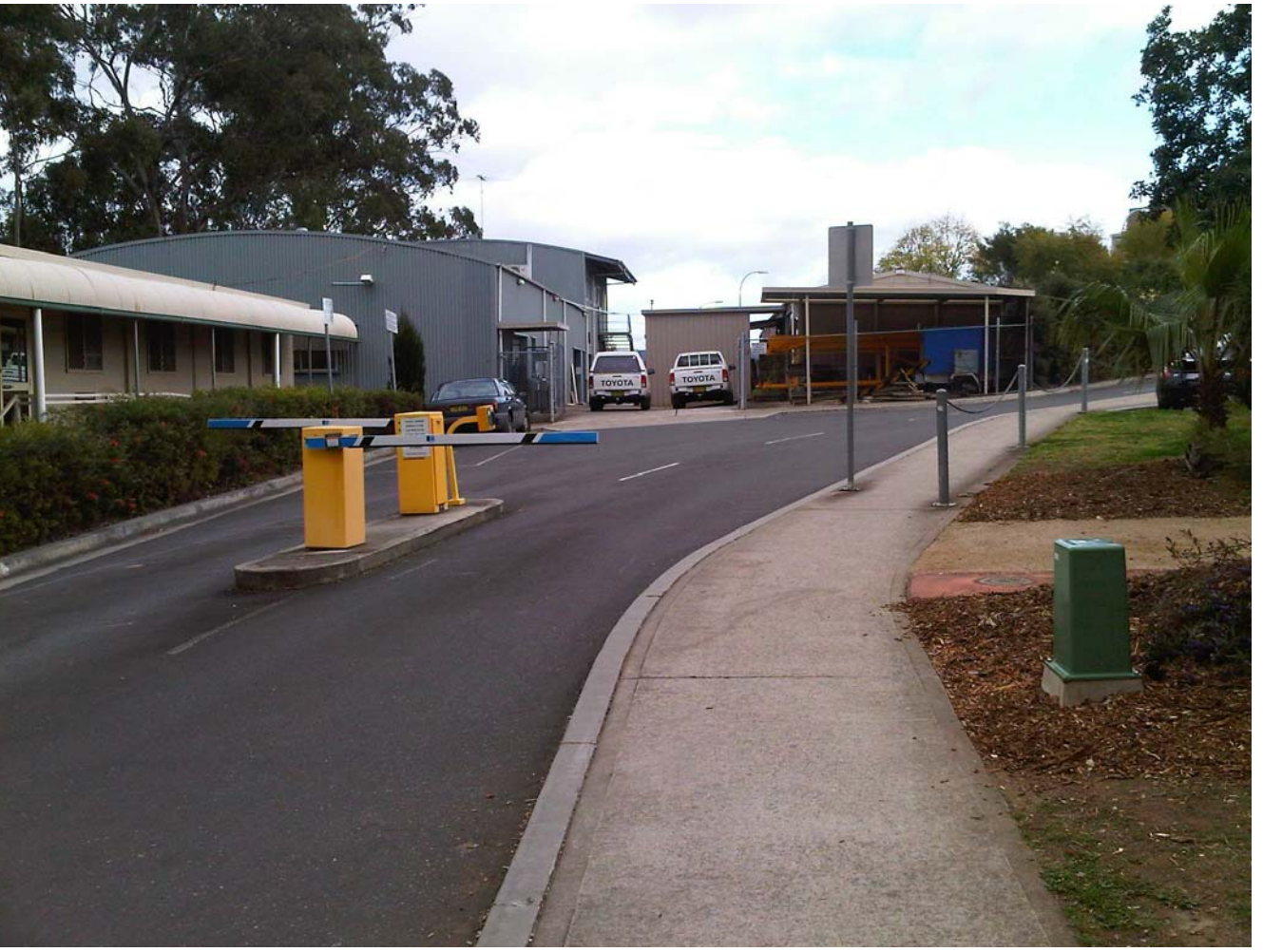
EXISTING SITE - VIEW 9
