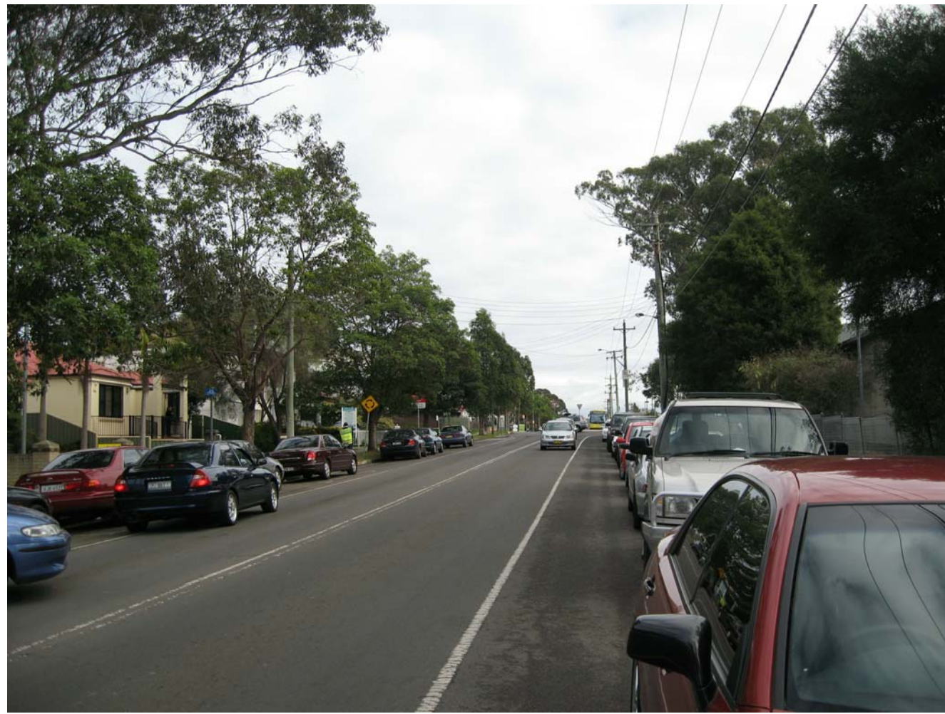
EXISTING SITE - VIEW 7
