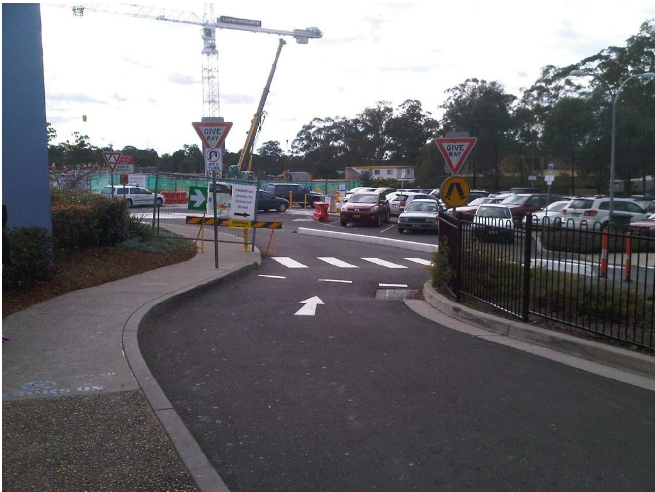
EXISTING SITE - VIEW 5
