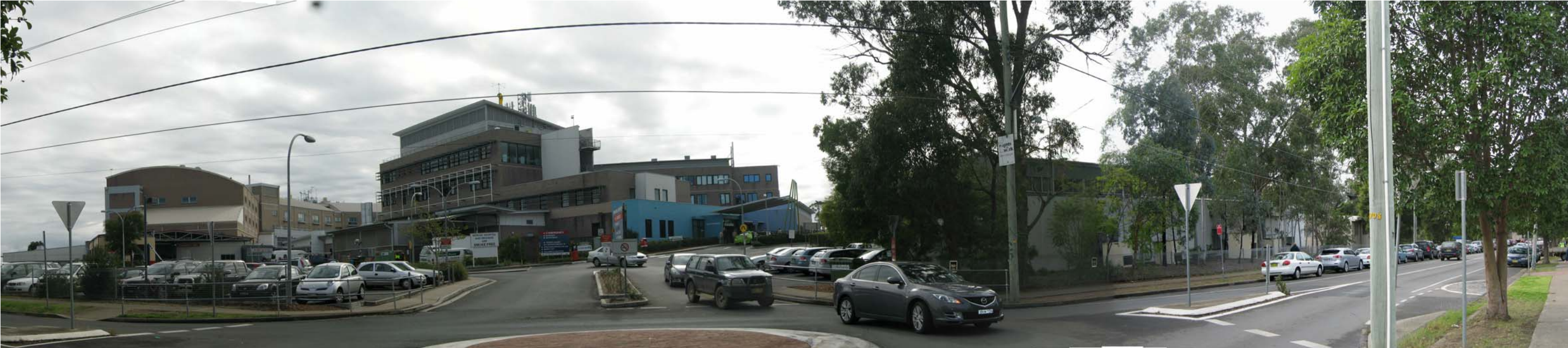
EXISTING SITE - VIEW 1
