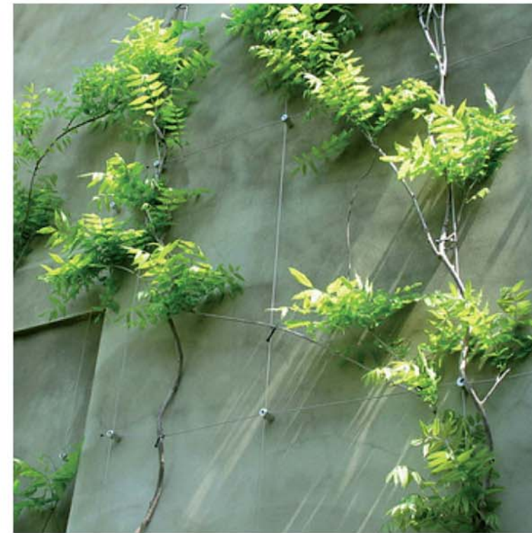
WALL PLANTING WITH METAL SUPPORTS (MF:02)
