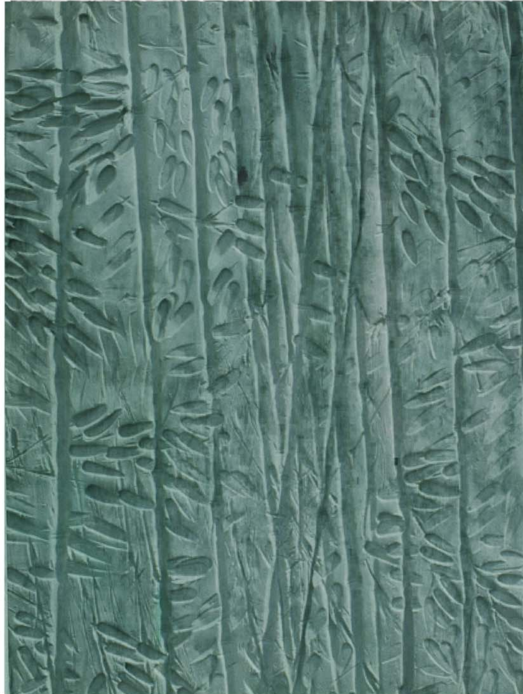
PRECAST COLOURED / TEXTURED CONCRETE COURTYARD FACADES (CE:01)
