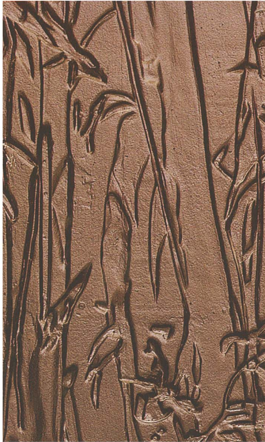
PRECAST COLOURED / TEXTURED CONCRETE COURTYARD FACADES (CE:01)
