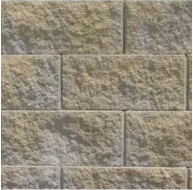
SPLIT FACE CONCRETE COURTYARD WALL (CE:01)
