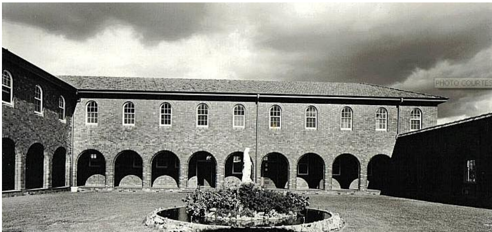
Figure 3 — The Cloisters in the 1960s showing the buildings that have previously been demolished as part of the approved residential development of the site that did not proceed.
