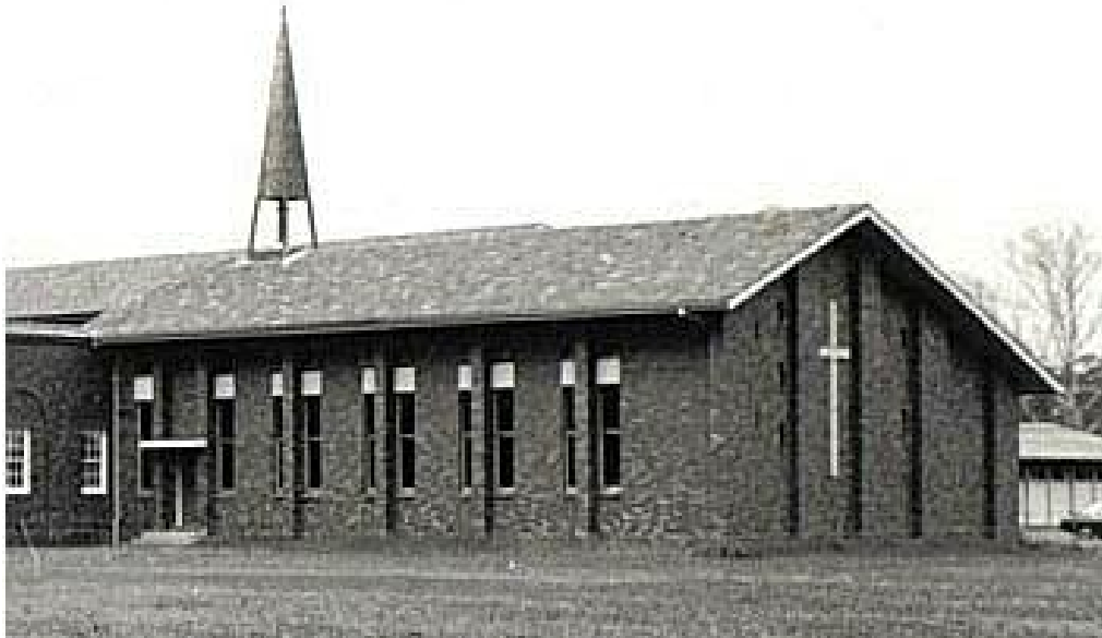
Figure 4 — The later, Post War Chapel structure that was erected on the western range of the cloister and has since been demolished.
