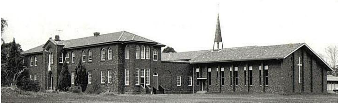
Figure 5 — The complex from the western side prior to the demolition of the rear wings and chapel.
