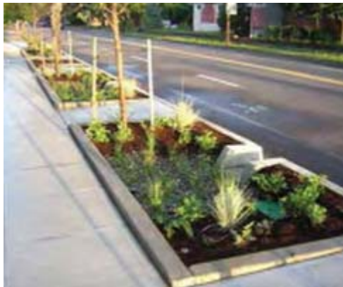
FIGURES 7.0, 7.1 AND 7.2 The WSUD measures proposed for the project include the use of bio-swales within the site to slow stormwater and treat it prior to releasing it into stormwater systems, as well as the use of low-flow, WELS-rated tapware and ultra-low-flow urinals.
