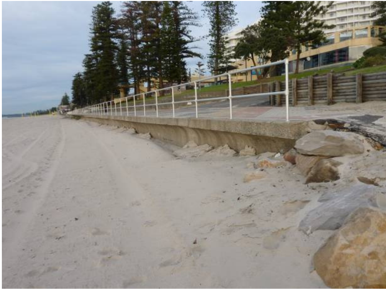
Photo 4: Wall at back of beach to contain sand
