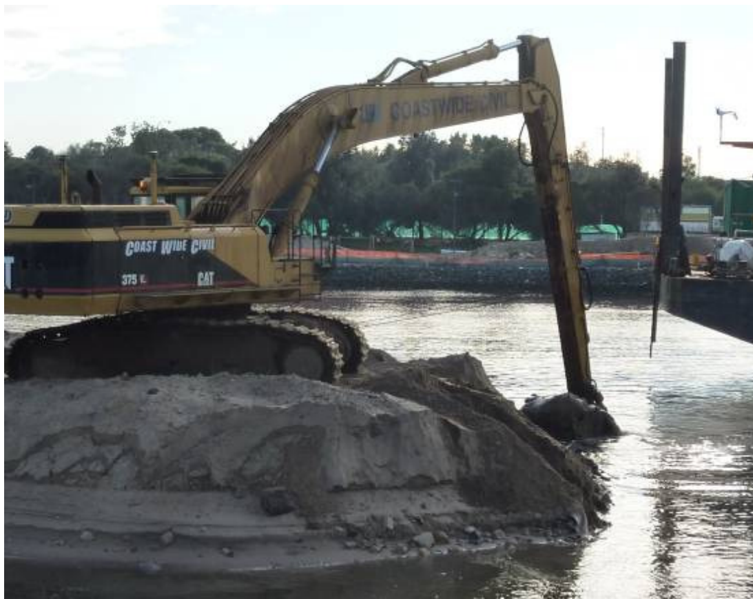
Photo 8 75 Tonne Excavator carrying out wet excavation
