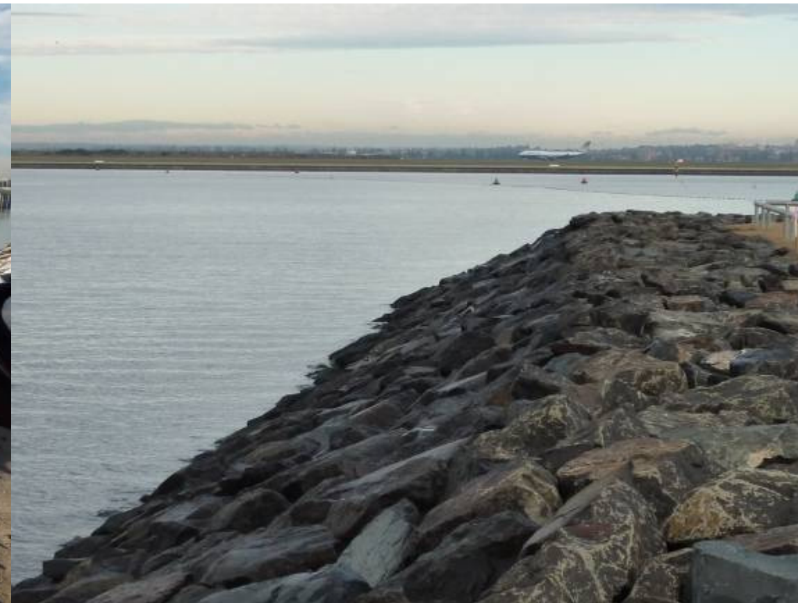
Photo 11: Relatively flat finished rock face achieved by the back of bucket of a large excavator.
