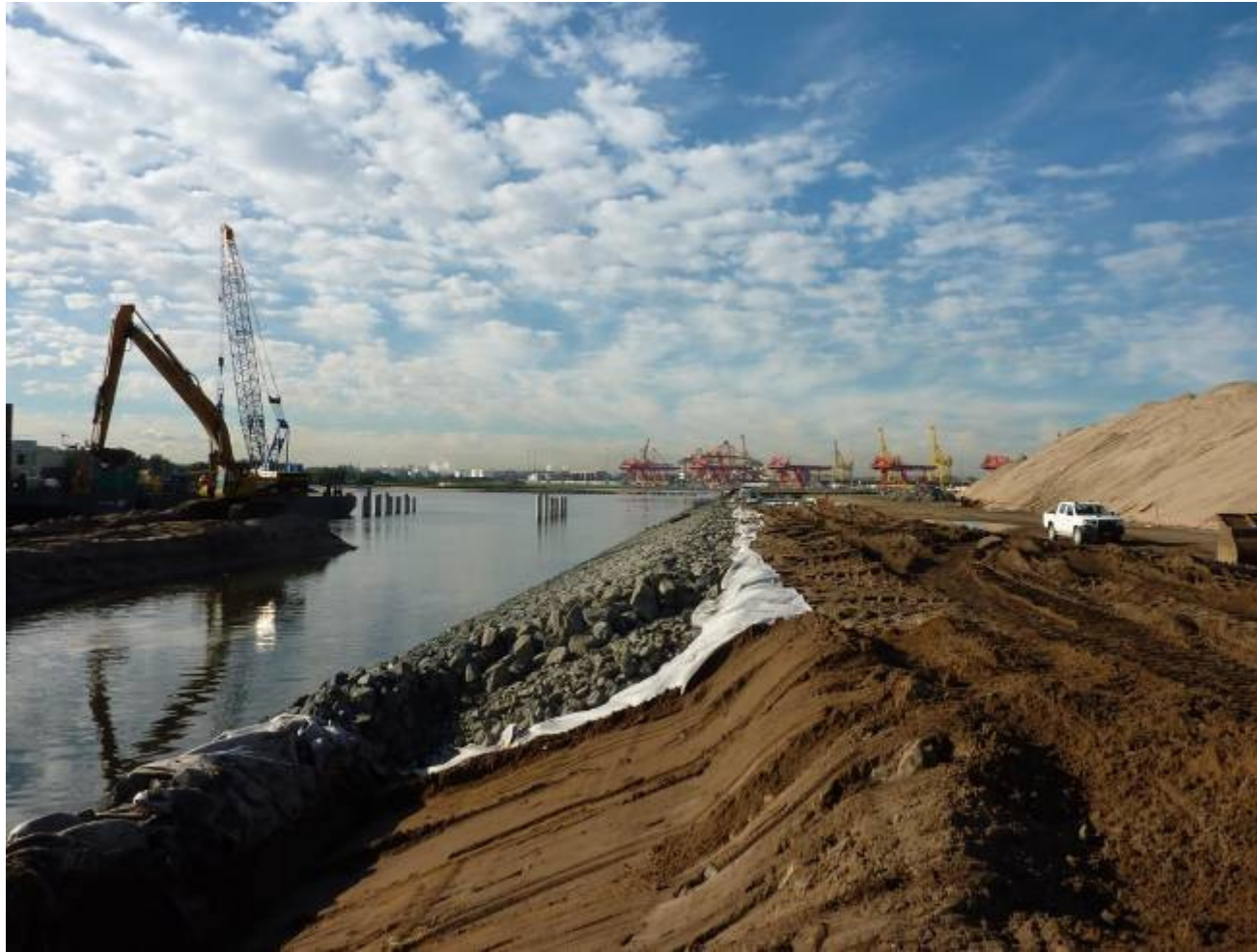
Photo 1: Rock Armour: Large Rock Armour Rocks over geotextile protection layer over geotextile on embankment.
