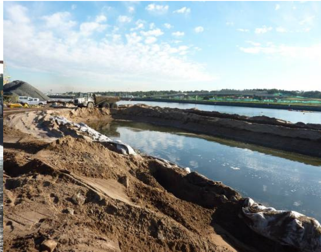
Photo 9 Typical bunded area for local dewatering
