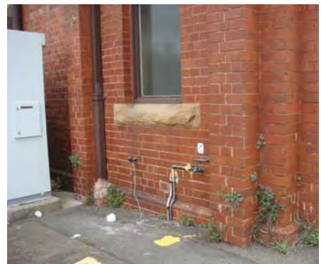
Fig. 3.16: Service penetrations through brickwork and weeds at base of walls.
