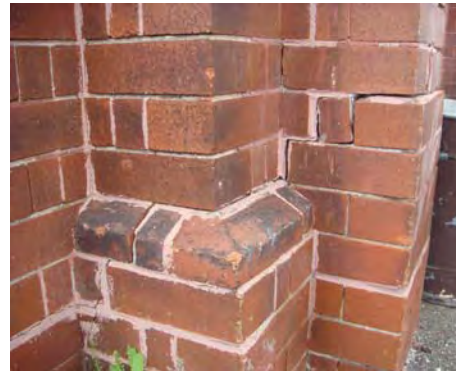
Fig. 3.14: Cracks in brickwork joints, evidence of inappropriate re-pointing with cement.
