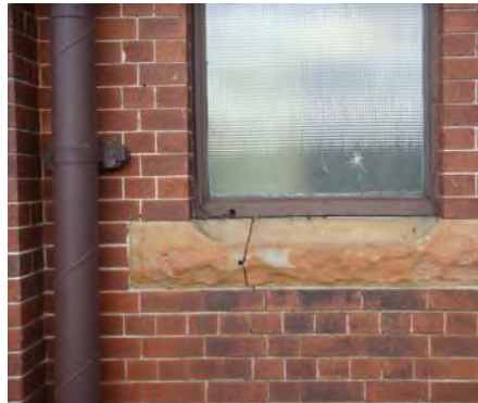
Fig. 3.13: Cracked stone sill and damaged glass
