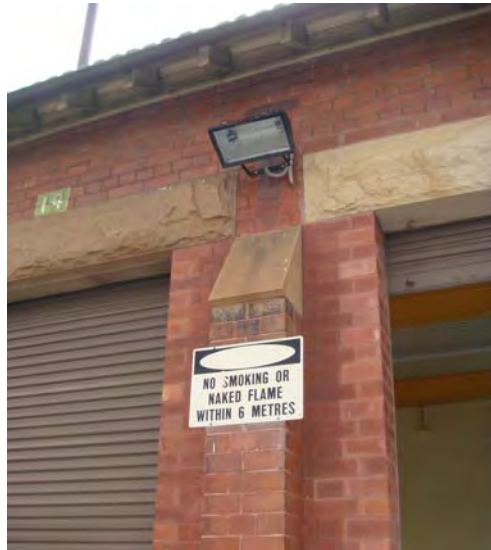
Fig. 3.11: The mark behind the light fitting is likely to be the remains of the original external crane. The changes to the brickwork at the openings, and the identifying '14' signage painted on the top left
