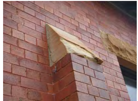
Fig. 3.12: Delaminating stone capping on a buttress.
