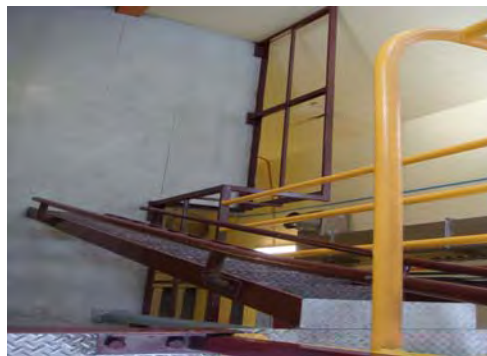
Fig. 3.9: Steel ladder and platform to pit below.
