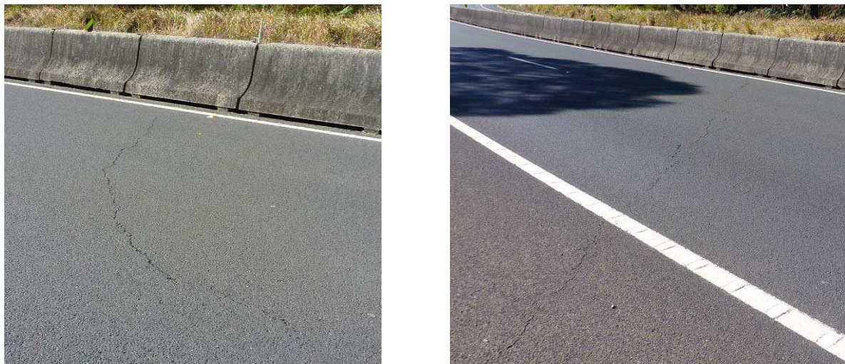
Figure 8 – Photos of subsidence related surface cracking from Mount Ousley Road inspection
