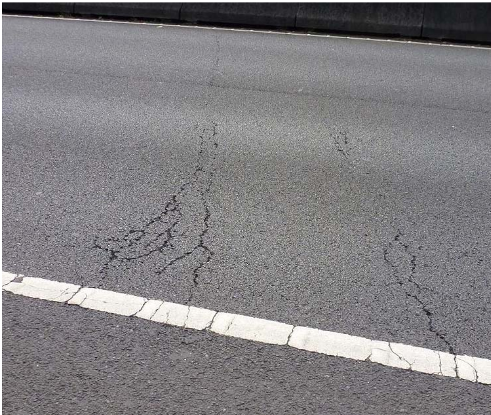
Plate 2A: View east at Survey Mark 24 on 9-10-12 showing existing pavement cracking in Lane 1 north and extension of crack into lane 2 (not present 21-8-12) and new crack south of original tension crack in Lane 1. The extent of cracking in this area has not changed over the past month since 4/9/12 (See Plate 1 Report 2)
