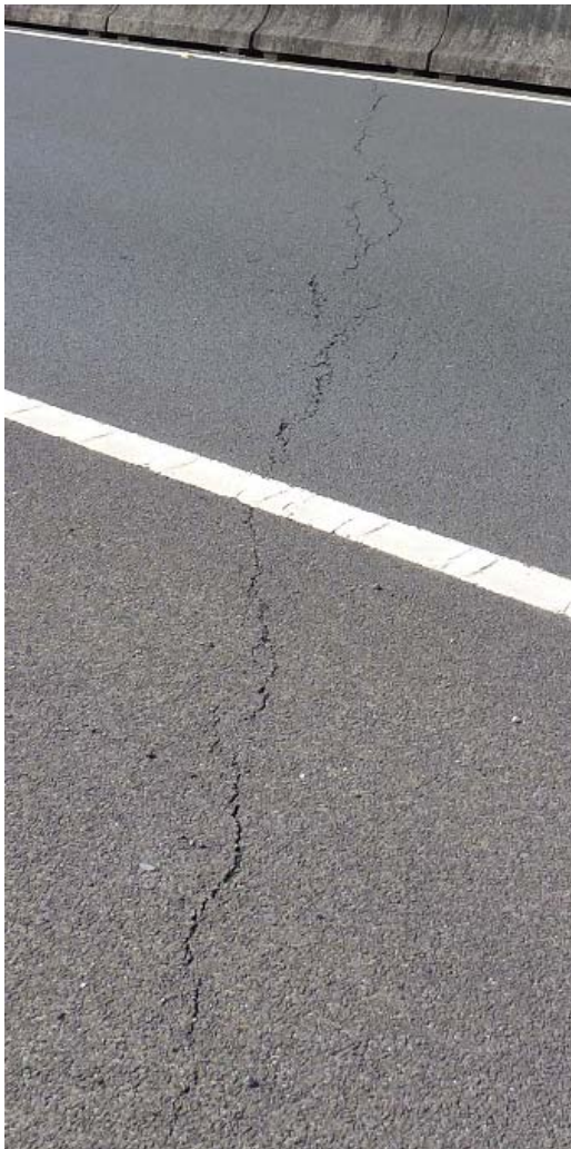
Plate 6 & 6A: Crack across NB pavement 4/9/12 left and 9/10/12 right
