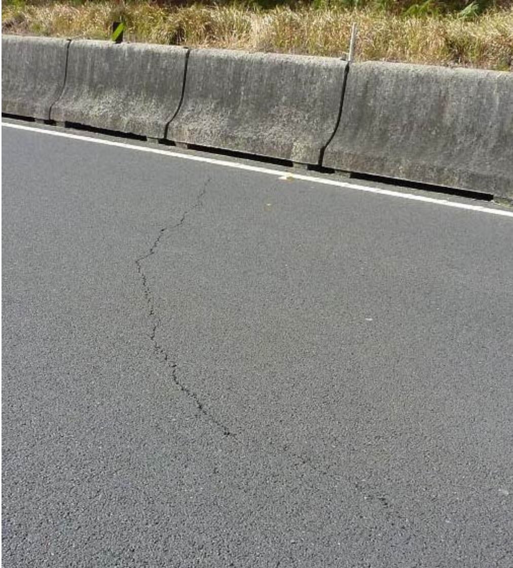
Plate 8: Tensile crack shown from 4/9/12 in Lane 2 North Bound at Survey Mark 48.0. Crack line extending across lane 2 SB at around 5- 10mm width no observable change on inspection 9/10/12
