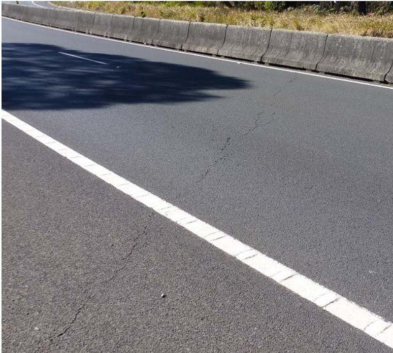
Plate 5: Photo from 21/8/12, shows diagonal crack across NB section of Mt Ousley Road at SM 46.10. Crack width approximately 2-5mm in lane 1 (kerb) and 5-10mm lane 2
