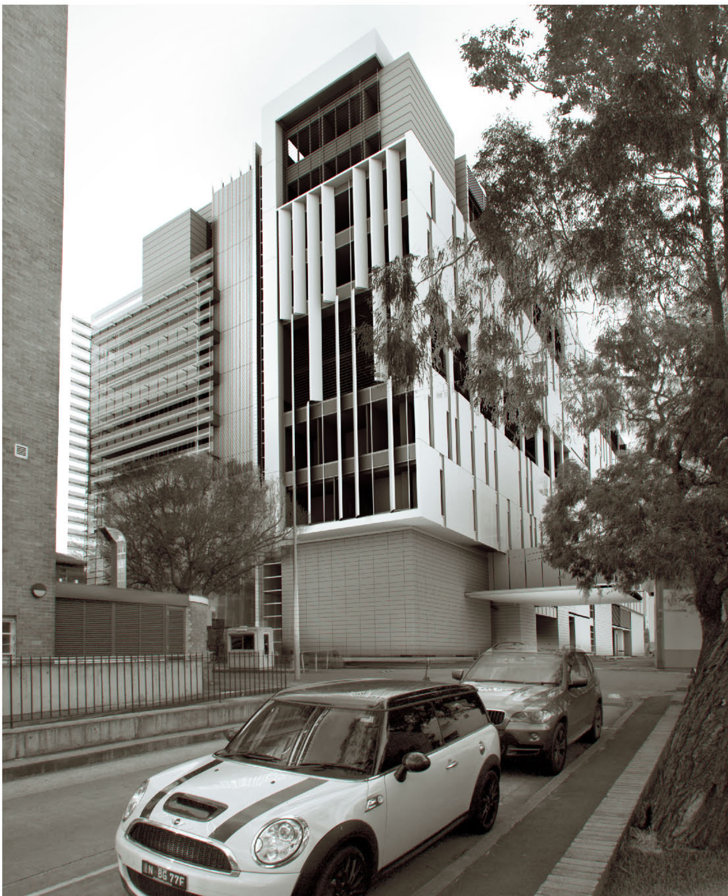
NORTH WEST VIEW
