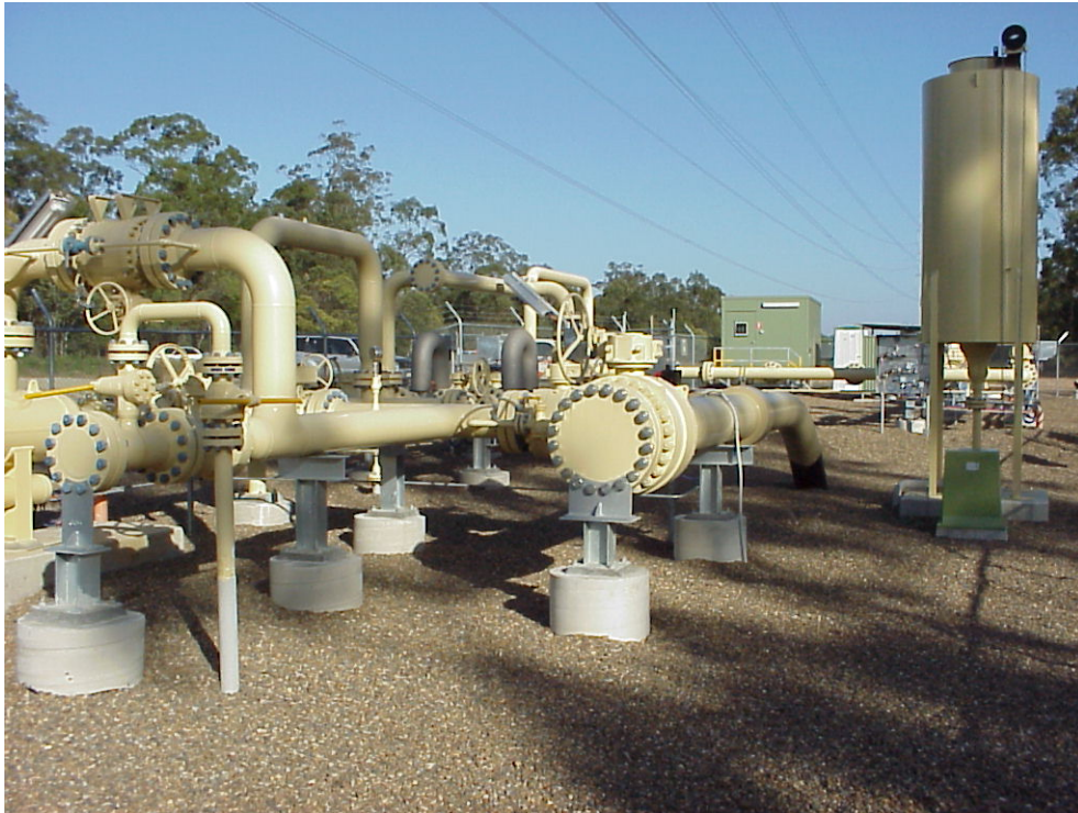
Plate 1 – Valve station, typical internal arrangement
