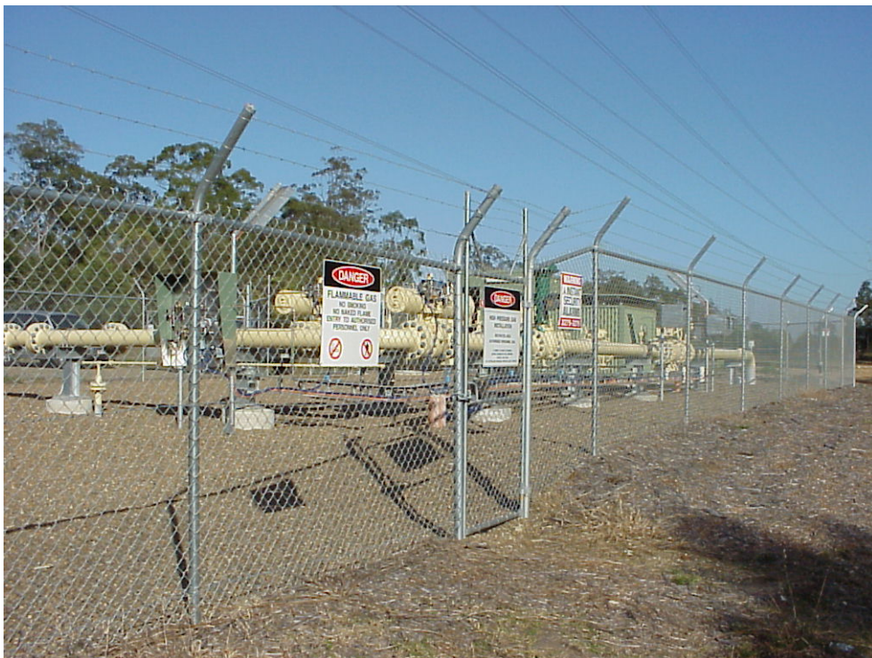
Plate 2 – Valve station, typical external arrangement
