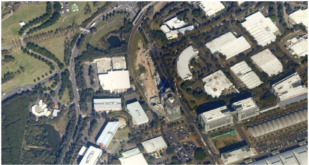
Figure 1b: Aerial Image of the Proposed Development Site (view from the North, facing South)
