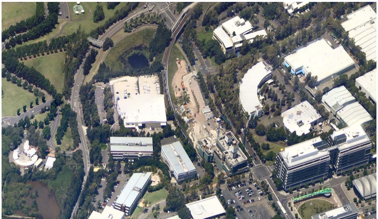
Figure 1c: Aerial Image of the Proposed Development Site (view from the north, facing south)
