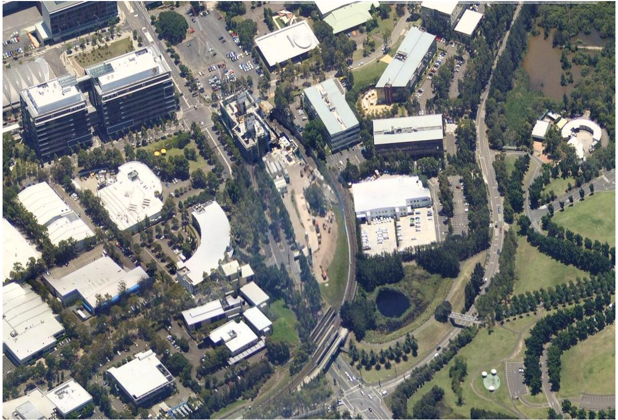
Figure 1b: Aerial Image of the Proposed Development Site (view from the south, facing north)
