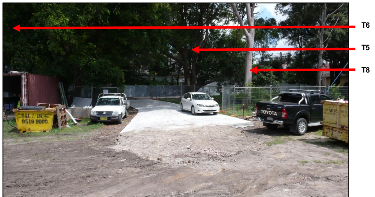
Photo D: Recently installed temporary construction Driveway between Tree 5 and Tree 6. More similar pavement is required adjacent Trees 5 and 6 for the Stage 1 and Stage 2 construction.
