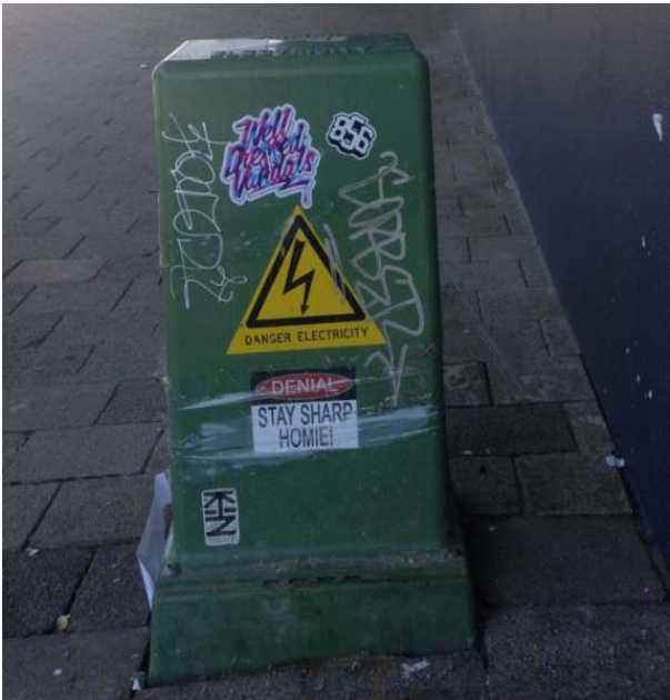
Figure 2: Ausgrid LV Network Pillar
