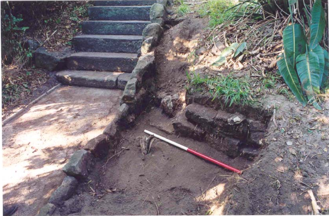
Figure 6: Lower section of path (near carpark) with retaining wall to west. Scale 1m.
