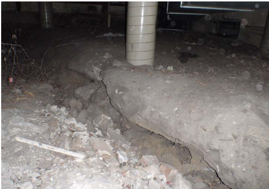
Photo 24: Piers below the Theatre showing erosional channel
