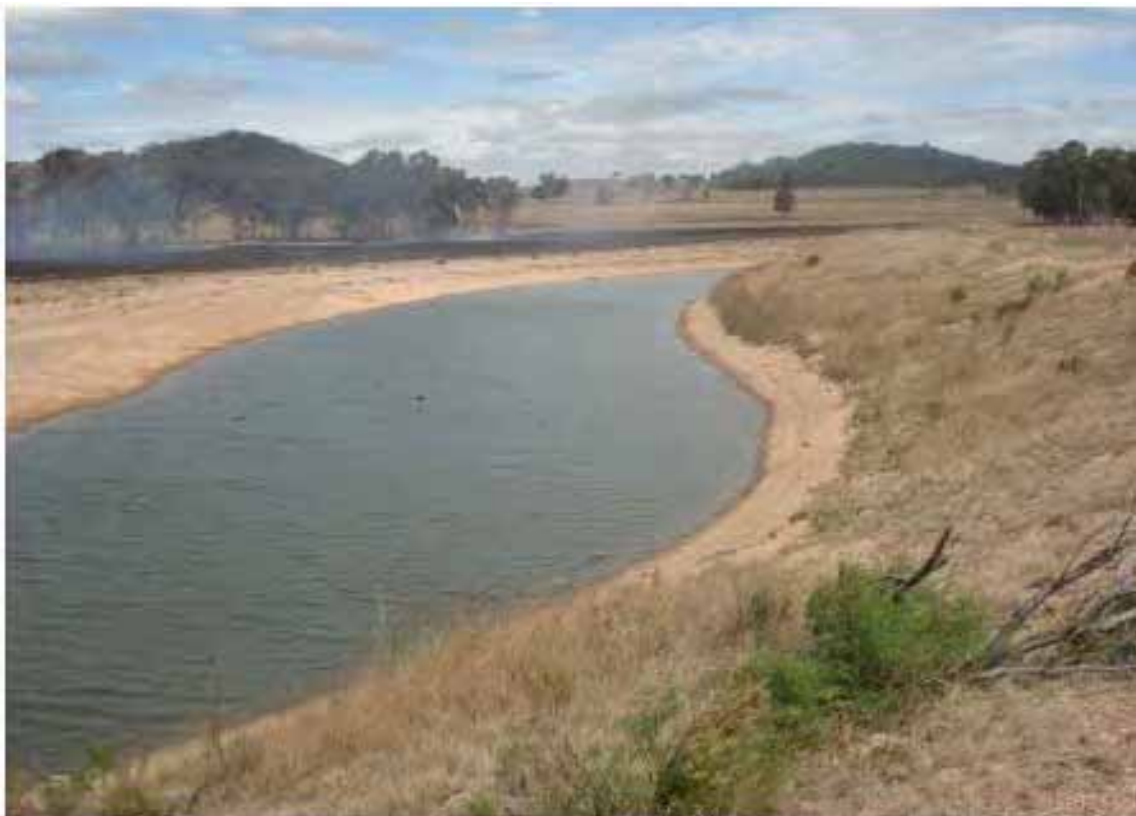
Photo 4-2 Sausage dam on Blackheath Creek
