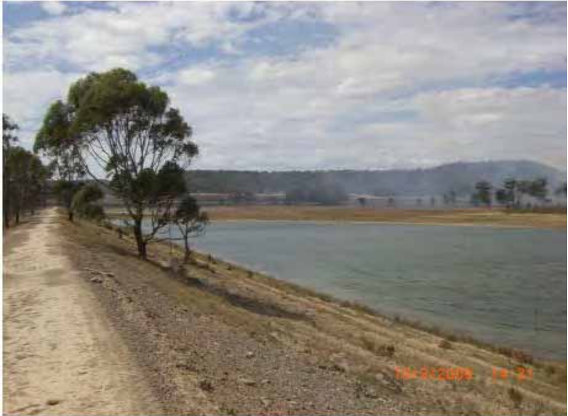
Photo 4-1 Catch water dam on Blackheath Creek
