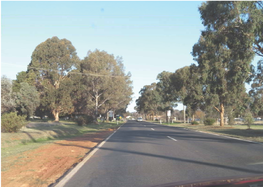
Castlereagh Highway, at Gulgong showing signs of shoulder edge drop off
