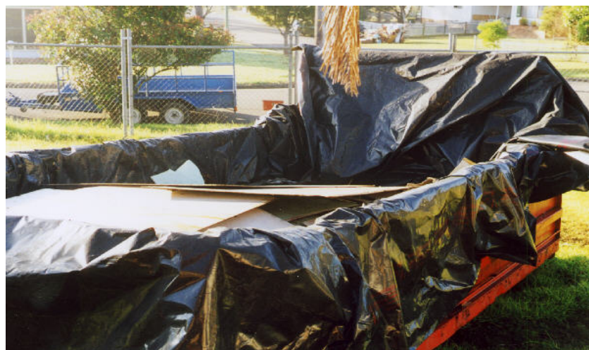
Photo 8 : Asbestos sheeting for removal off site
