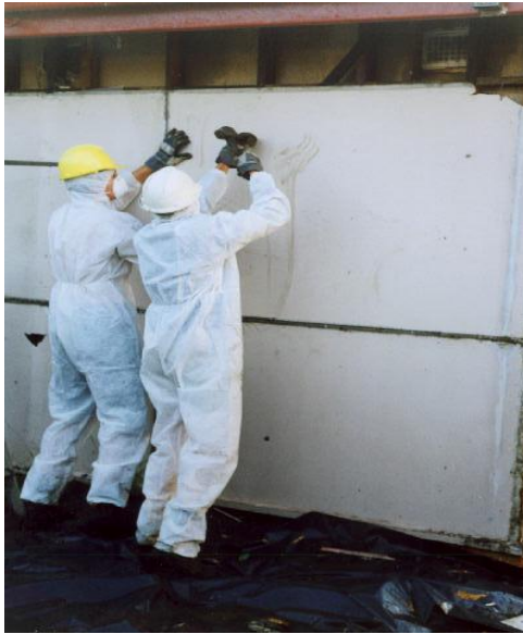
Photo 6 : Asbestos sheeting removal – preparing for sheet removal
