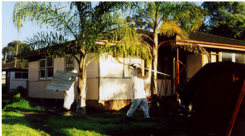
Photo 7 : Asbestos sheeting removal
