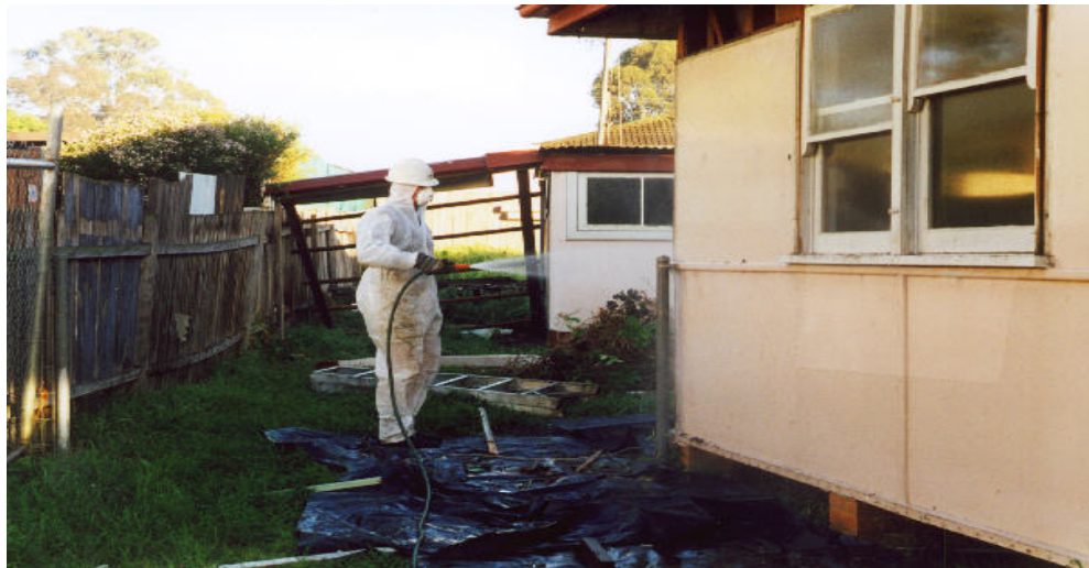
Photo 5 : Asbestos sheeting removal – wetting down the surface
